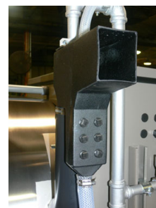
Safe chemical injection
