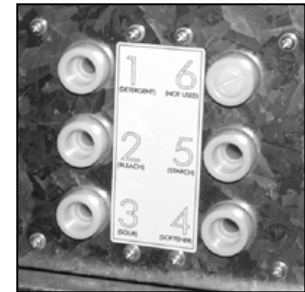
Safe chemical injection
